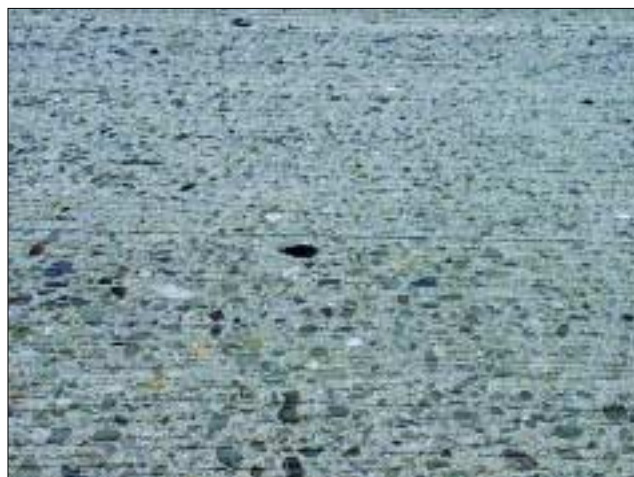
Figure 2. Route 101 surface after diamond grinding.
