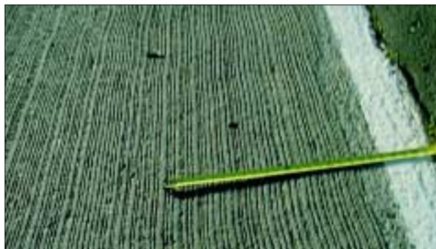
Figure 1. Longitudinal grooves of Route 101 at the test segment.
