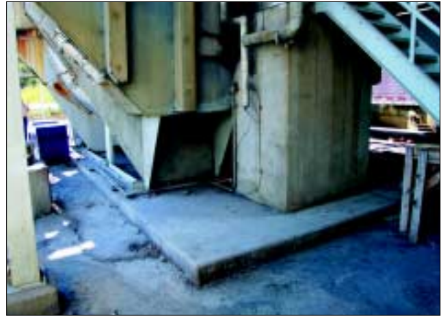
Figure 4. Embedded foundation, fan outboard bearing pedestal.
