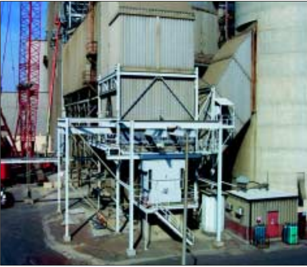
Figure 2. ID fan, motor end.
