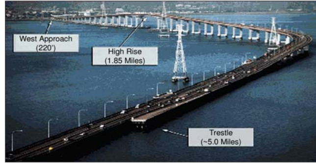
Figure 2. San Mateo Bridge.
