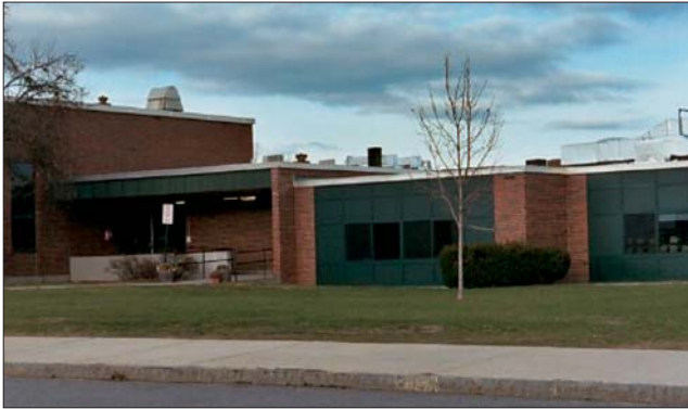
Figure 4. Front façade after sound insulation modification.
