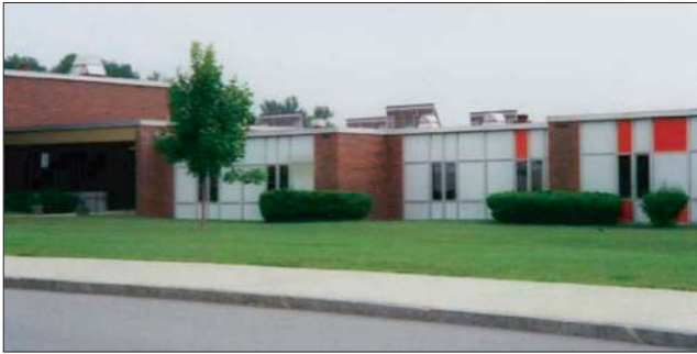
Figure 3. Front façade before sound insulation modifications.
