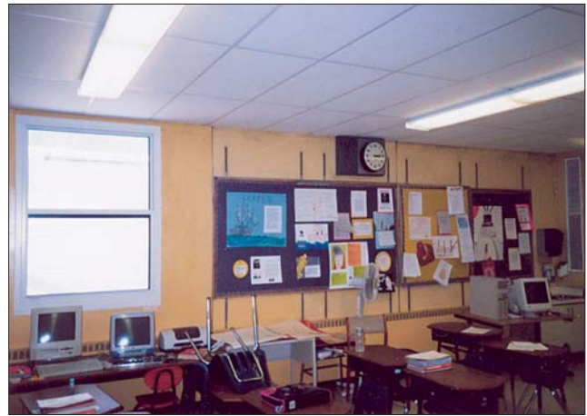
Figure 2. Exterior wall of C-wing classroom.
