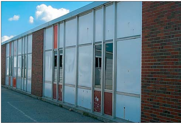
Figure 1. Exterior curtain wall at A- and B-wings before modifications.
