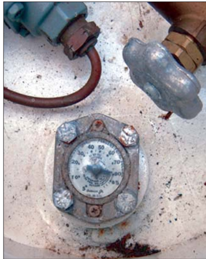
Figure 1. What gives here? The gauge indicates nearly 80% liquid charge remaining.
