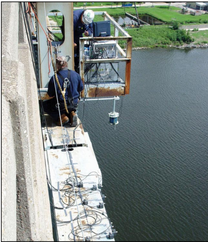
Technicians installing AE sensors.
