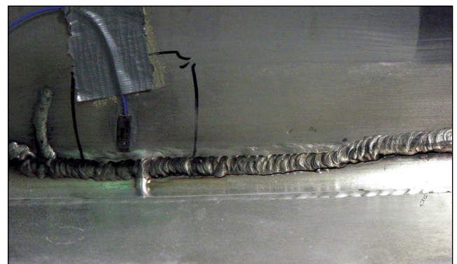
Figure 10. Piezoelectric gage mounted to failed vessel.
