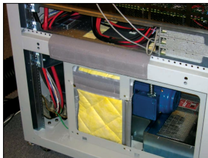
Figure 2. Blankets placed around motor.
