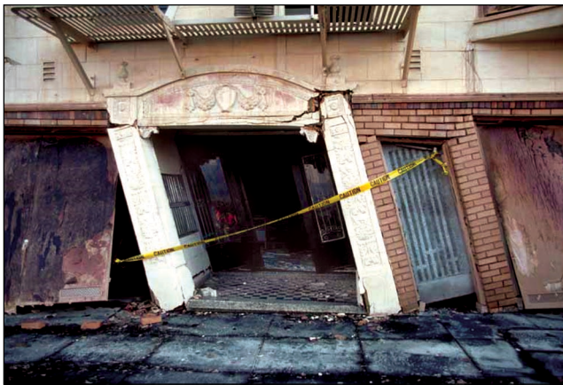
Figure 11. Earthquake damage to apartment building in San Francisco's Marina District.
