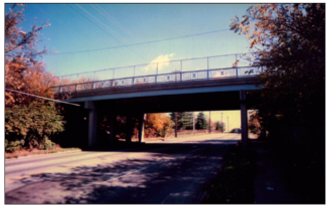
Figure 1. Seymour Street Bridge.
