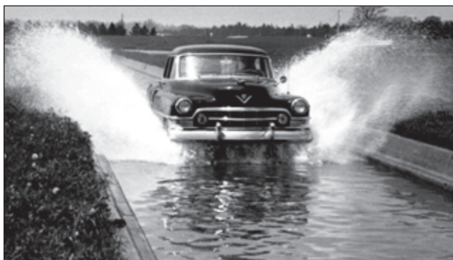
Bathing an early 1950s Cadillac in the Water Trough to verify integrity of brakes, ignition, starter, generator, door seals, and splash deflectors. Don't ever try this with your English sports car!
