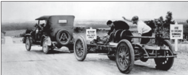
An early towed dynamometer measured the actual tractive effort delivered by an automobile.
