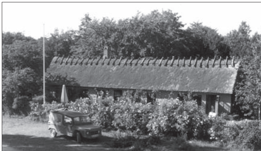
Per Brüel's summer house on Anholt.
