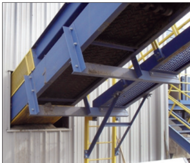
Figure 9. Shredder conveyor opening.
