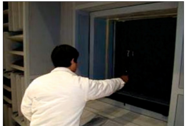
Figure 15. Wuxi Jixing's sound transmission facility.
