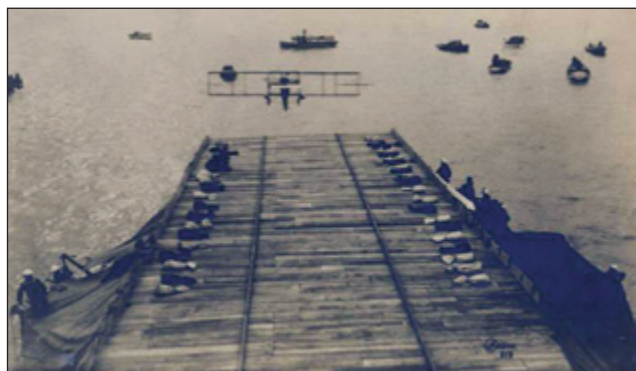
Figure 13. Note the "Tail Hook" arresting system; a hook attached to the landing gear used to catch a series of ropes attached to sand bags. January 18, 1911; first shipboard landing of a Model D Curtiss flying boat by Eugene Ely on a 120 x 30 ft wooden platform on deck of the USS Pennsylvania (photo courtesy Naval Historical Heritage).
