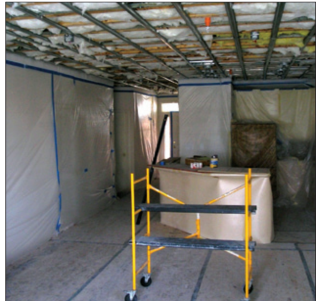
Figure 8. Existing ceiling demolition and spring isolated ceiling installation.
