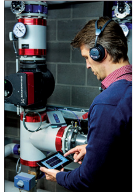
LMS SCADAS XS connected to pump sensors being remotely monitored using an LMS Smart Scope and LMS 3D Binaural Headset.
