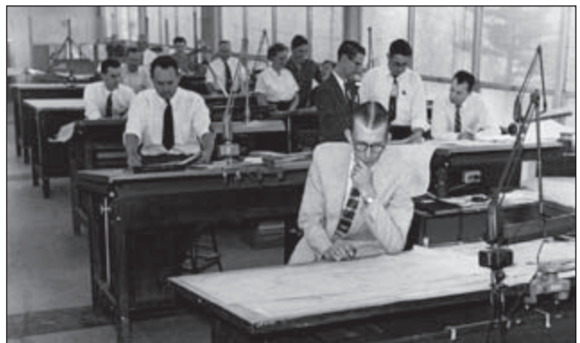
MB Electronics engineering and drafting room, circa 1955.
