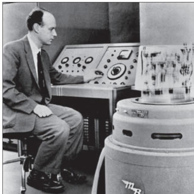
Don Vanorsdall runs swept-sine test, September 1959.
