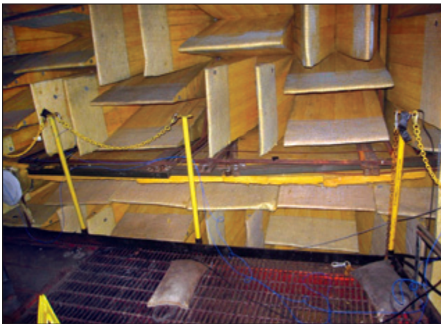
Figure 4. Anechoic side of original STL opening with removable wedge sections in place.
