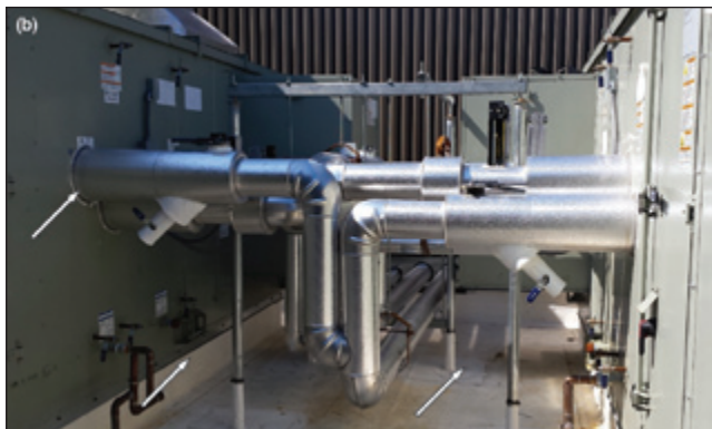
Photo 3. Pipes and ducts are rigidly connected to units and roof with potential vibration and noise transfer.
