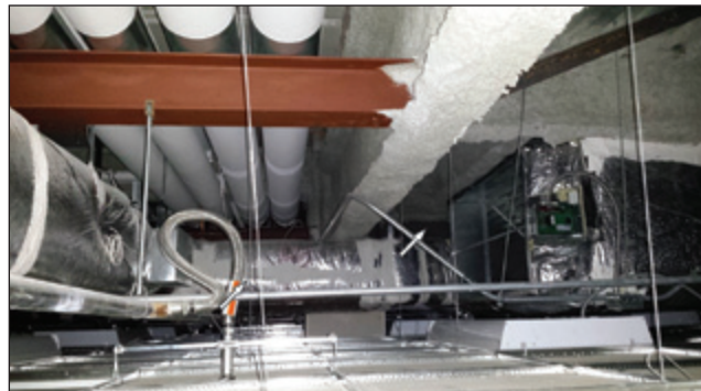
Photo 1. Return duct elbow connected directly to the fourth-floor units located directly above sensitive spaces.
