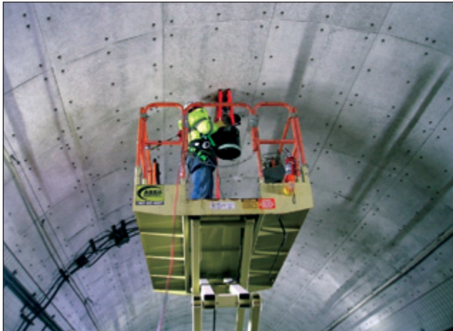
Figure 5. Attaching RSS to tunnel ceiling.
